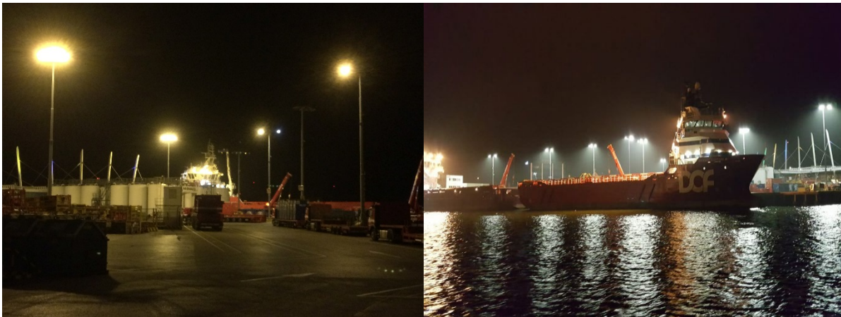
The left image shows the conventional lighting, the right image shows energy-efficient, smartly controlled, LED lighting.
